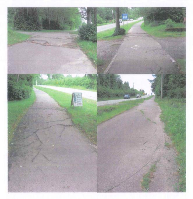
Bike Path Pavement Damage – tree roots that have lifted pavement surface creating hazards. Location is between Willowbrae Road and Millstream Subdivision along Tofino Ucluelet Highway.
